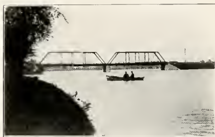
Old Independence Bridge
